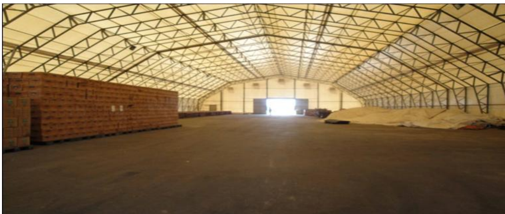
Photo – Storage facilities for food aid commodities are expensive infrastructure investments, even some of the temporary facilities such as the Rubb Hall storage warehouse. Clean and neat facilities and properly stacked commodities are the start of sound storage practices and key to integrated pest management.
