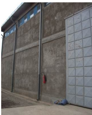
Photo no. 3: Save the Children Warehouse in Adama, Ethiopia showing gaps underneath the door
